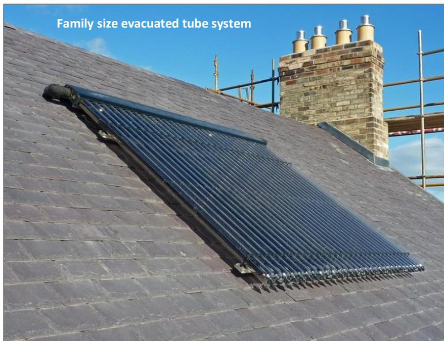
You will need a southerly facing roof, wall or piece of ground for the panels or evacuated tubes and new hot water storage tank.
