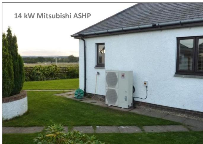
Heat pumps are not suitable for all properties. They work more efficiently with a low temperature heating system and are therefore suited to **energy efficient, well insulated buildings**. There is however scope for flexibility in the system design – heat pumps can be used with radiators and can be 'docked' with existing heating systems to assist the heat pump during very cold weather. In order to establish the right size of heat pump for your home, a detailed heat loss assessment is required.
